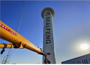
[Dealfeng](#) has successfully completed their 24m x 4m flettner rotor on shore, a major breakthrough in Dealfeng rotor technology, and also represents a large step forward in wind-assisted technology for China. By installing these rotors, ships can achieve a 5%-20% saving in fuel consumption. Dealfeng has specialized in R&D and manufacturing of marine energy-saving equipment for vessels for many years, and the rotor systems has received LR AiP certification.
